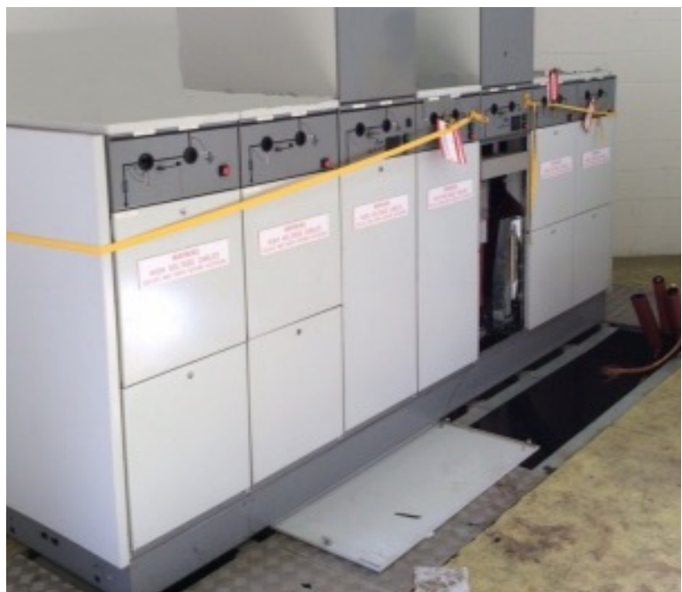
Figure 14 – “Barrier “out” method for the erection of a barrier on totally enclosed switchgear
