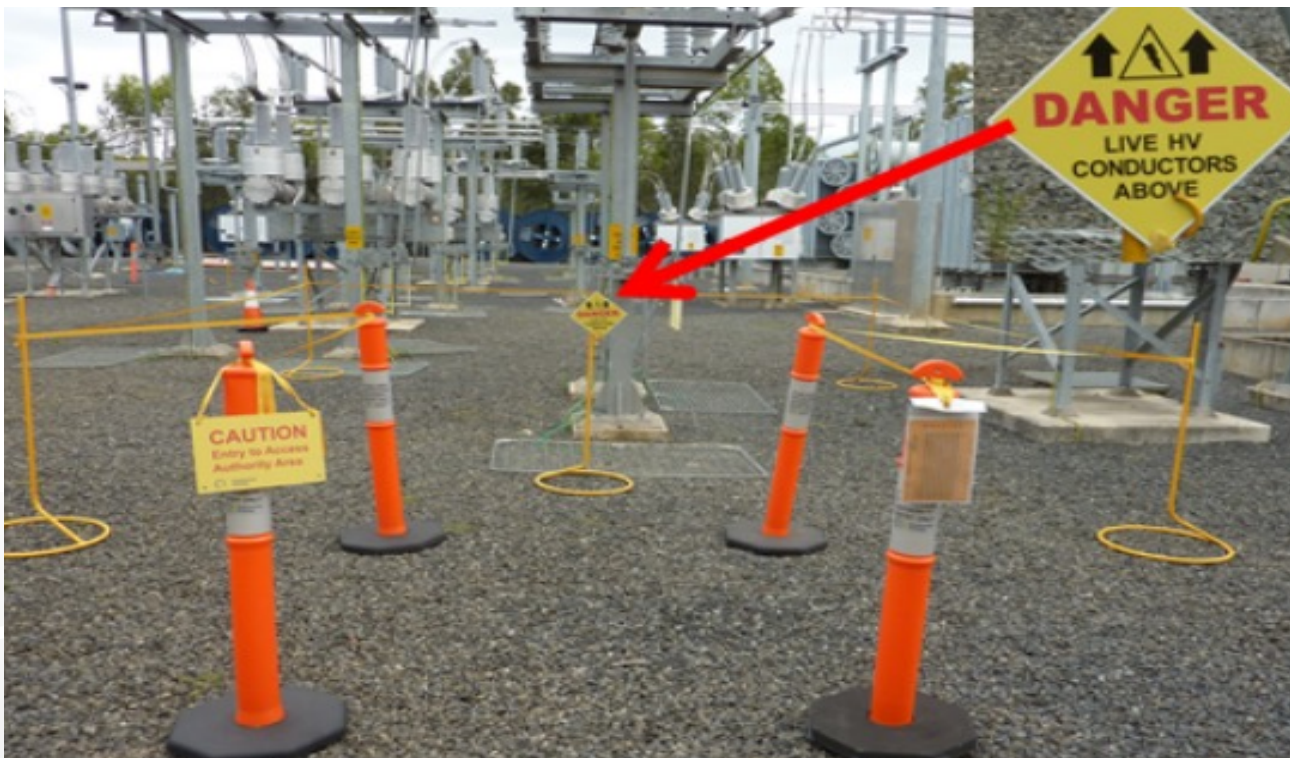
Figure 12 – Barrier “in” method for the erection of a barrier in a substation showing “DANGER live HV conductors above”
