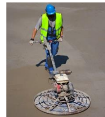
Trowelling Machine (Helicopter)
